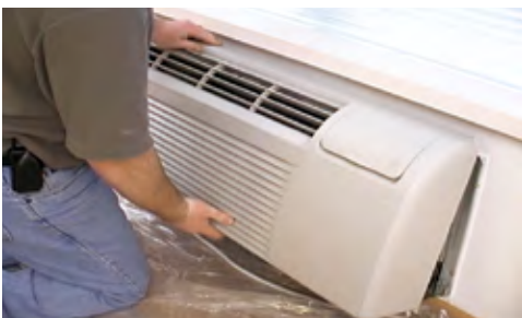
Step 2. Remove the room-side front cover of the unit.
