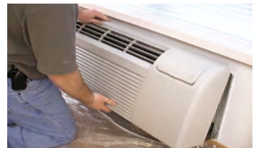
Step 8. Reattach the cover, then plug in and turn on unit.
