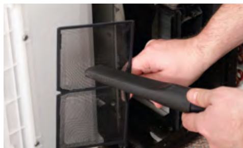
Step 4. Vacuum accumulated dust and dirt off the filter.
