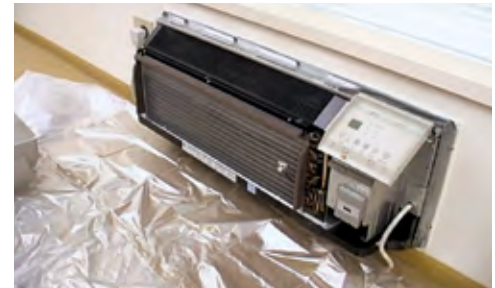
Step 7. Replace filter and slide the unit back into sleeve.
