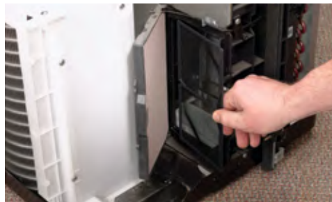
Step 3. Pull the unit from the sleeve and remove the filter.
